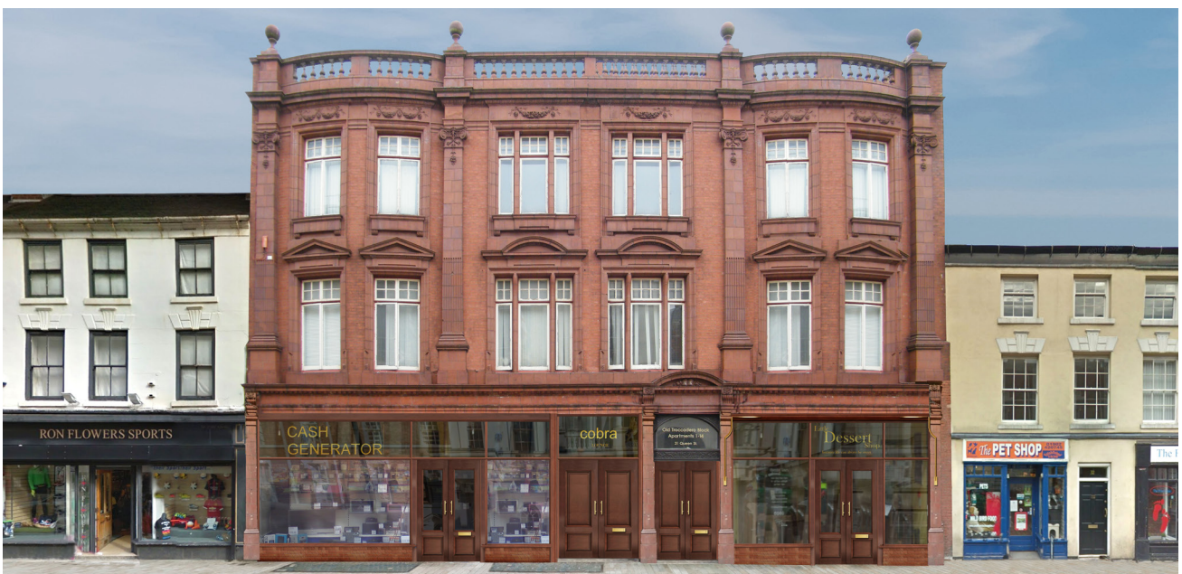
The former Trocadero Building, 29 to 31 Queen Street
