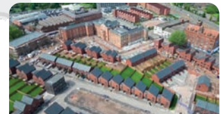
whg Affordable Housing Development.
