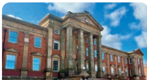
whg 55+ Affordable Housing Wellbeing Scheme Development.
