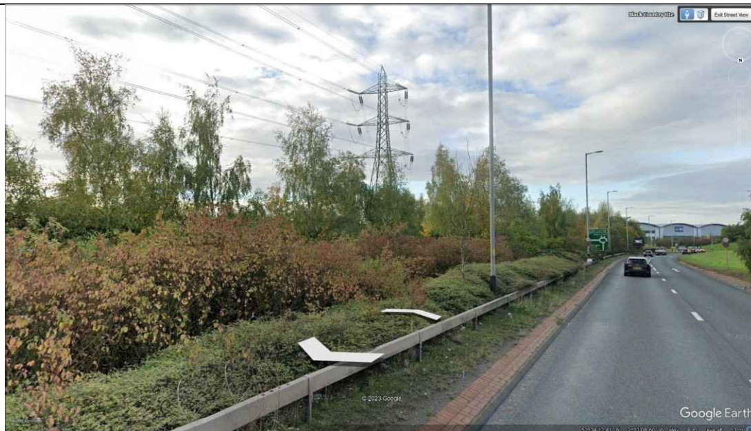
Location - Black Country Route, approaching Lunt Junction westbound Lampost 22
