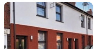
Retrofitted Council properties, managed by Wolverhampton Homes
