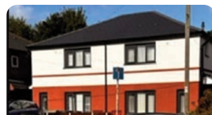
Retrofitted Council properties, managed by Wolverhampton Homes.
