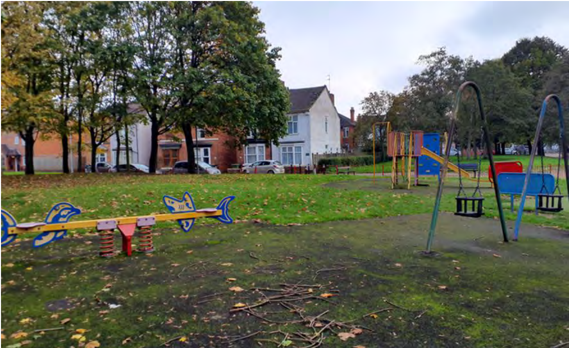
Tired surfacing and equipment, Leicester Street Open Space (ID 64).
