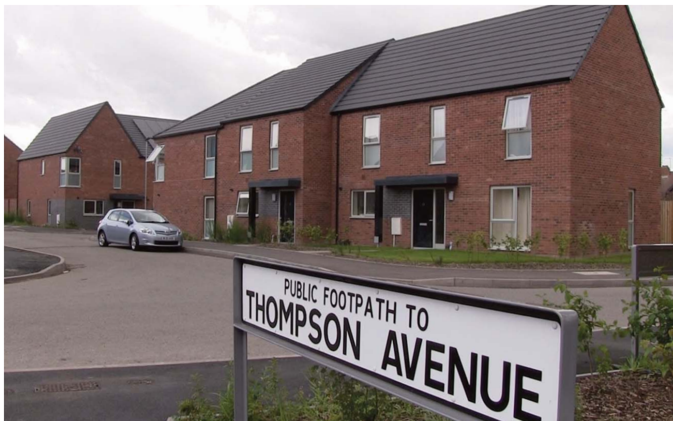
The first council houses to be built in Wolverhampton for thirty years at Thompson Avenue
