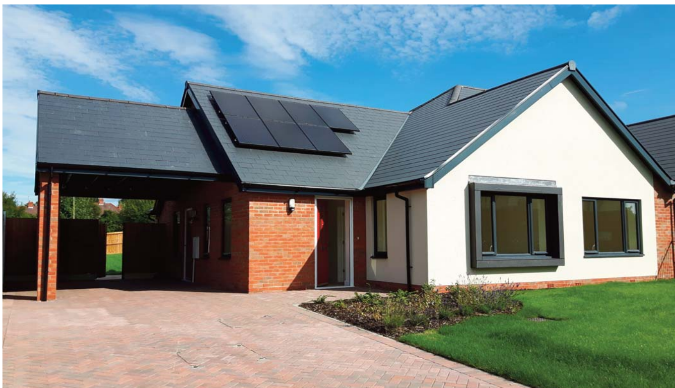
Properties built for the Care and Support Specialised Housing Scheme at Fifth Avenue
