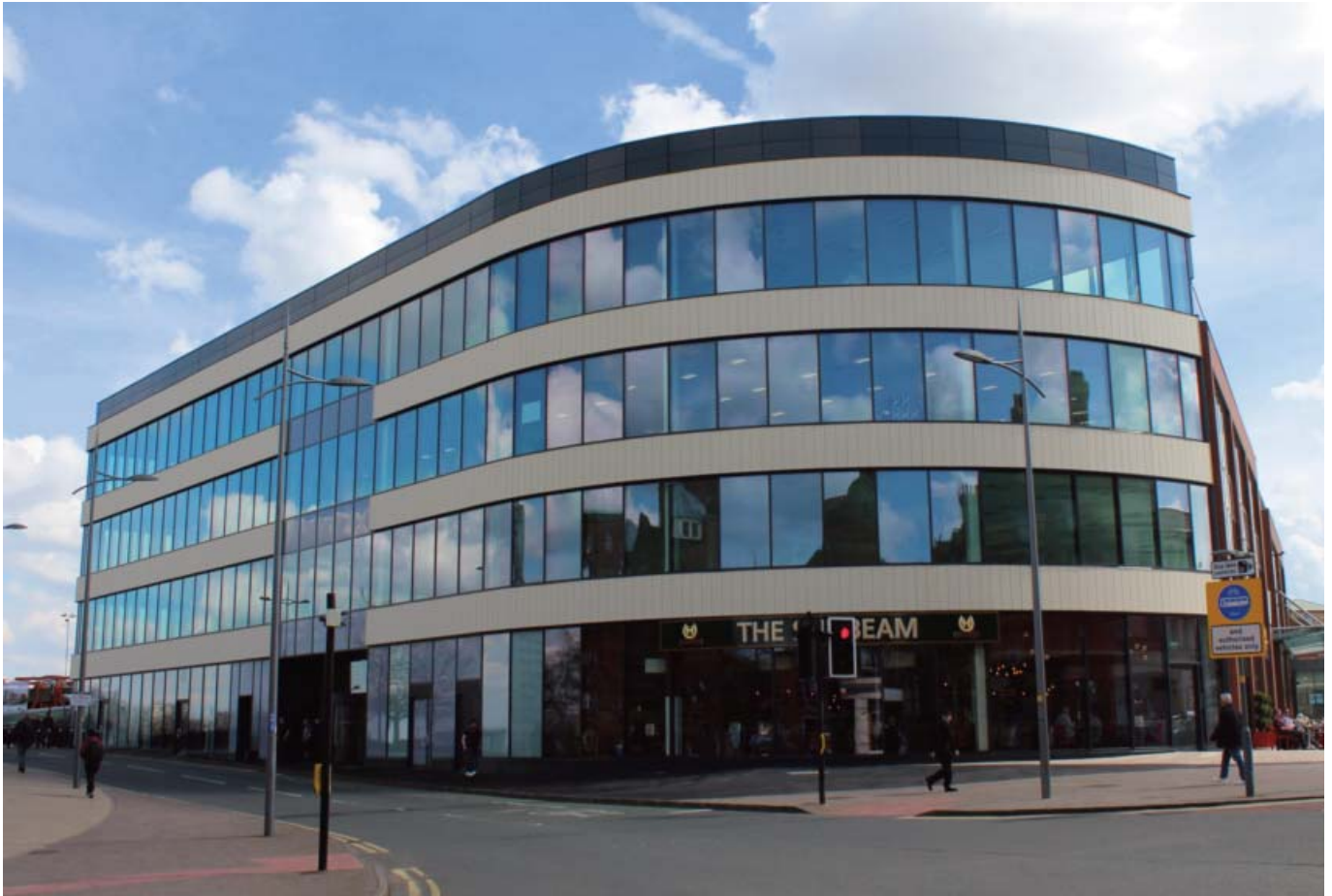
The New i10 Development on Railway Drive, Wolverhampton
